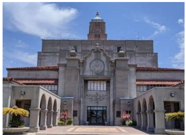
MWD Weymouth Admin Building, – MWD October 13, 2025
