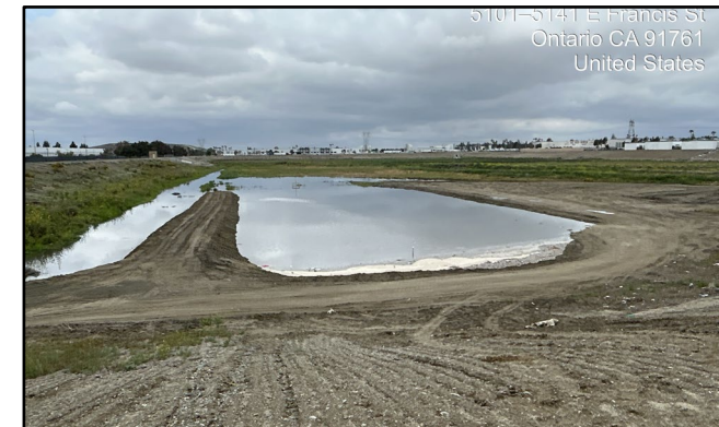
Completed Basin at Wineville
